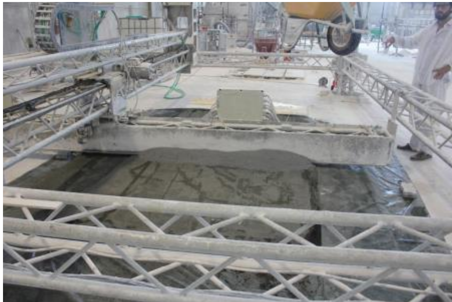
Sand leveling procedure using the trowel
