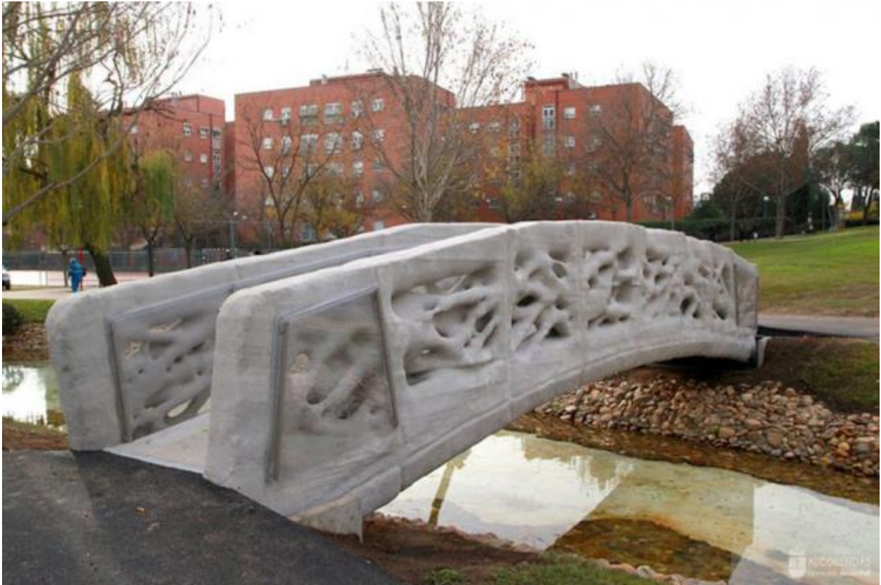
First 3D Printed bridge in the world located in Madrid, Spain
