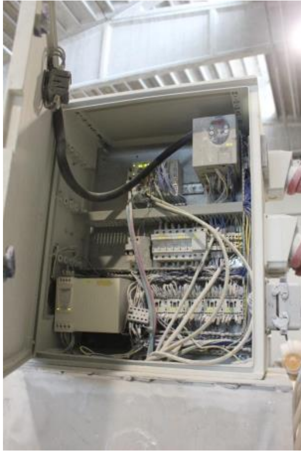
Programmable logic controllers mounted on top of the printer
