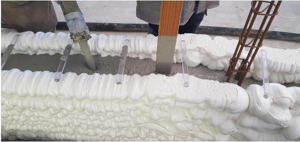
Concrete pouring in between the polyurethane formwork.
