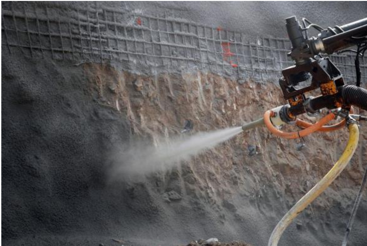
Shotcrete for stabilizing ground (notice also the addition of a reinforcement steel mesh in the top part of the surface)
