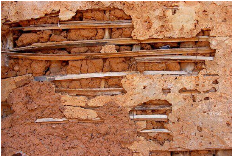
A deteriorating earth wall
