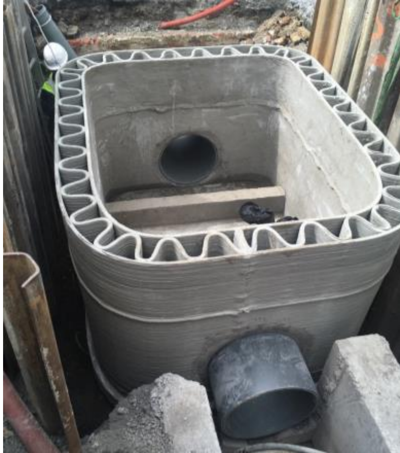
A sewage over-flow shaft, installed in Lille province, France.
