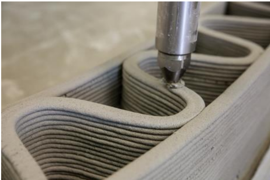
An XtreeE print, with very thin even layers, and a finely grained surface
