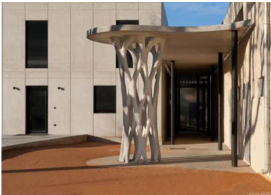
A complex-shaped column, the first 3d printed structure installed at a public school
