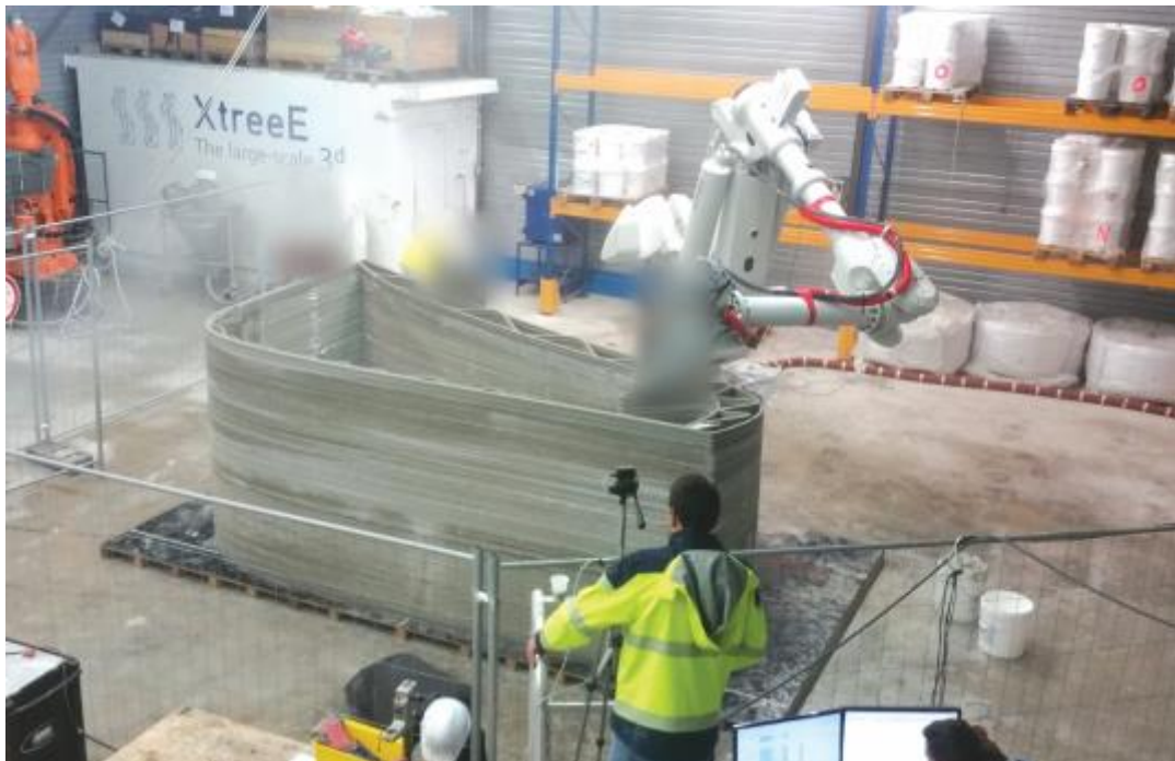
The Xtree printing technology in action
